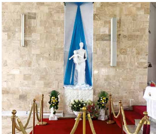
The main PA is formed from couplings of SR-S4L and SR-S4S speakers
